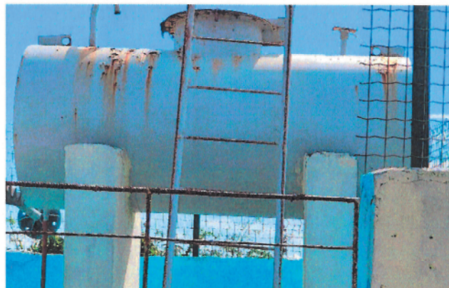
fig.4 Diesel tank
