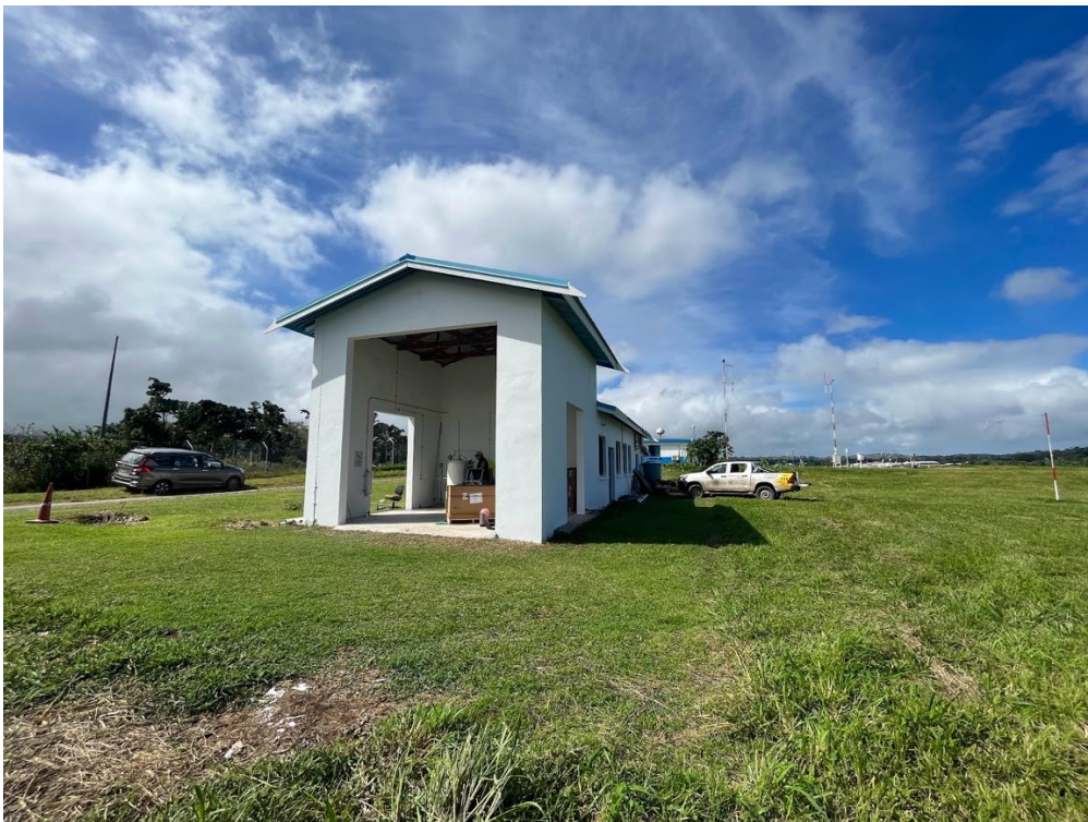
Figure 5 Bauerfield Balloon Shed – subsequent to refurbishment.
